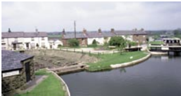
Two photographs of an English canal dry dock of similar construction to the Solovki dry dock. Note the stop planks for keeping the water out, and the keel blocks on which the boat sits. Water is allowed to drain away into the canal below the two locks on the right of the bottom picture. This dry dock suffers from leakage through its walls when full, resulting in water entering the cellars of the houses. Dock walls of this type are always difficult to keep watertight.
