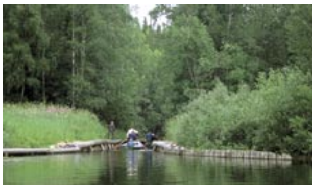
The rebuilt southern entrance to canal K8.
