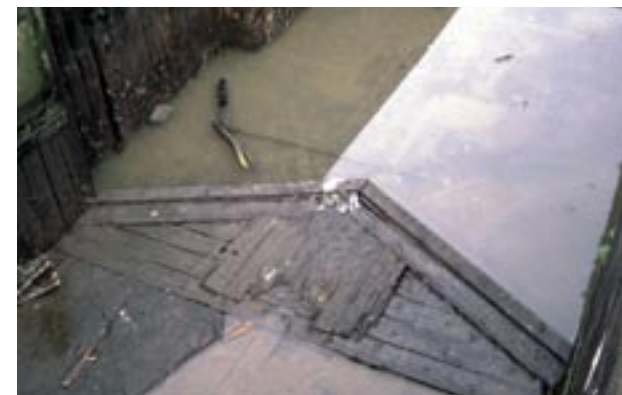
A photograph of a wooden gate sill on an English canal lock. Details vary from canal to canal, as does the angle of the mitre. However, they are usually around 140 degrees. The gates on the dry dock should have a sill similar to this to form a watertight seal.
