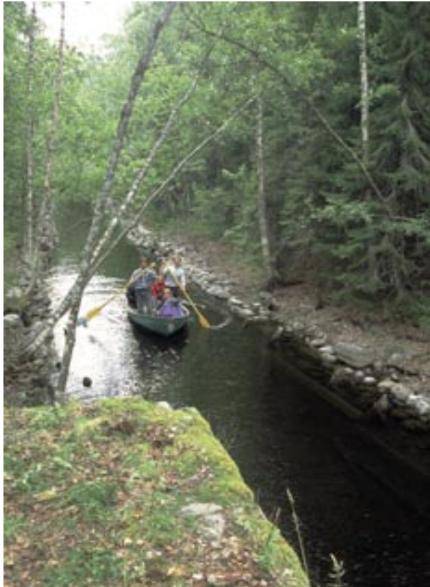
Canal K5 viewed from Sluice 1 looking to the south. The water level appears to have been raised and covers the bank protection.
