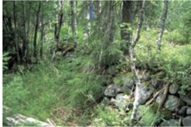
Dam D1 was constructed to raise the water level in the lakes now forming the northern section of area No.1. Together with the construction of canals K9 & 10, this allowed the waters of these northern lakes to be diverted southwards and to improve the supply for the new hydro-electric station.
