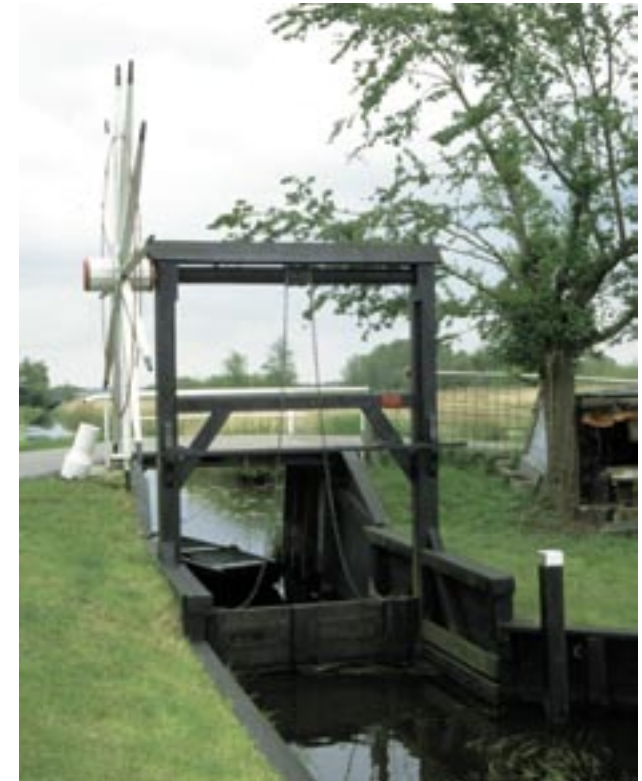
A restored wooden lock in Holland, typical of the many which were used for land reclamation, drainage and navigation.
