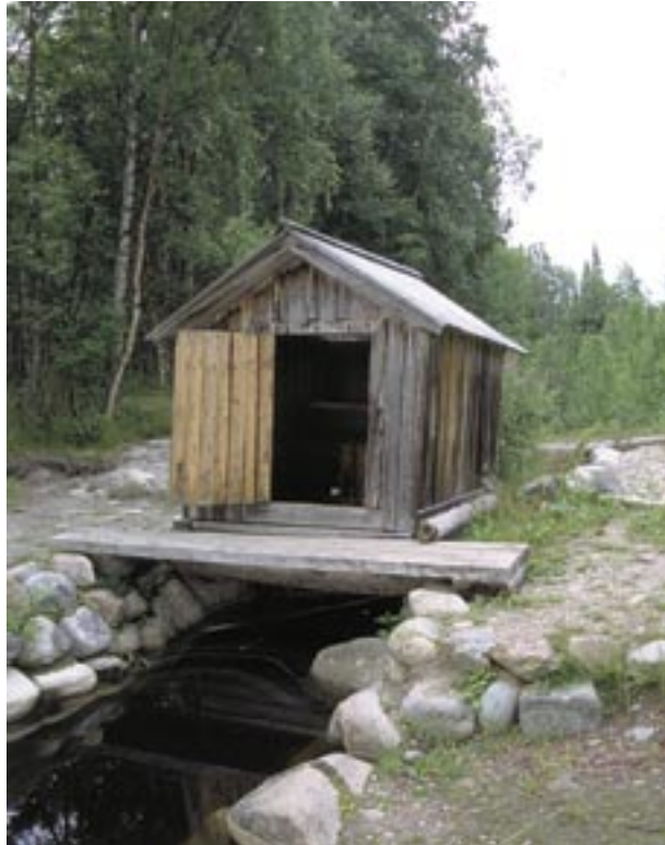
The house for sluice 2 which controls water supply to canal K1 and the Saint Lake.
