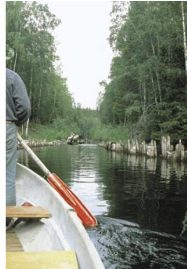
Unrestored canal K10, built in the early 20 th century, looking north. There are several types of wooden bank protection to be found on the navigable canals. Some have continuous vertical or horizontal planking whilst others use a wooden framework for stabilising random stonework.
