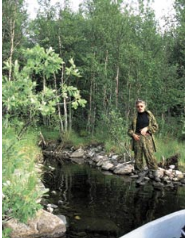
The western end of canal K3, one of the water supply canals. The sides of the canal have been protected with stone to prevent erosion. Wood was also used for this purpose.
