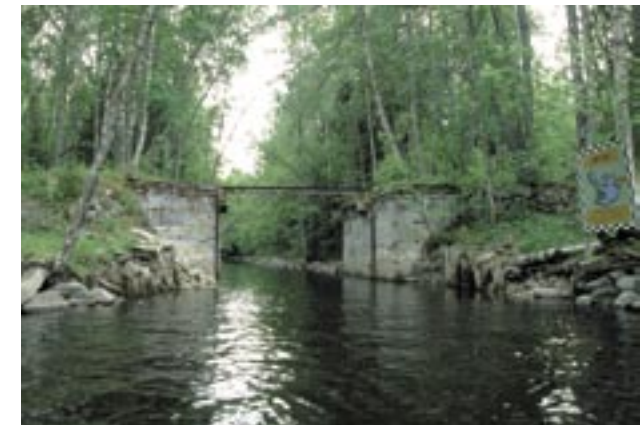
Sluice 1, above, was built to control the water supply for the hydro-electric station. The gate and gate-raising mechanism have been removed.
