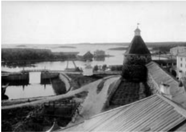
A view of the dry dock from the monastery, taken around 1910. Note the type of wooden fencing around the dry dock and supply basin, and the bridge over the dock entrance.
