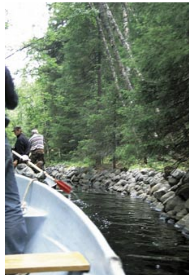
Near the middle of canal K6. The stone bank protection is typical of several of the island's navigable canals.
