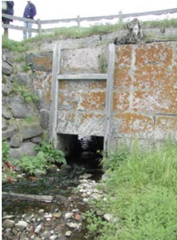
The remains of the water supply control sluice in the basin to the north of the hydro-electric station. The wooden frame is fixed against the dressed stone wall suggesting that it may have been added later.
