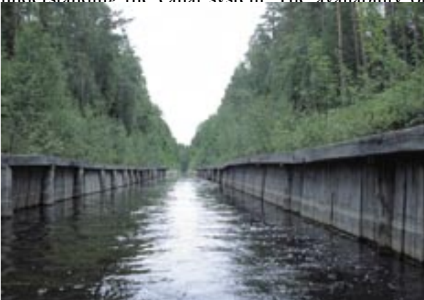
Part of the restored section of canal K7. This end of the canal has wooden bank protection, while random stonework is used at the other end.
