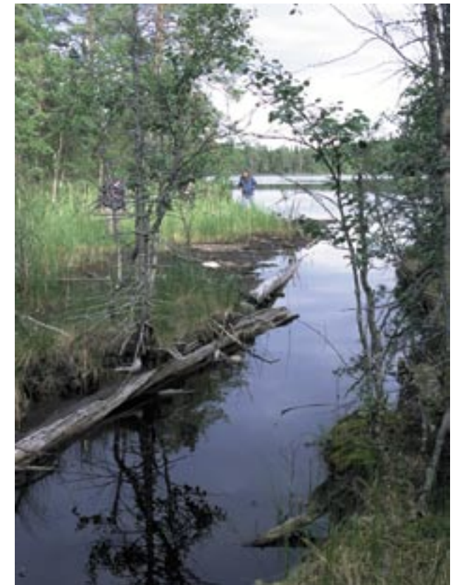
The eastern end of canal K3, one of the 16 th century water supply canals. Logs have been used to protect the sides from erosion.
