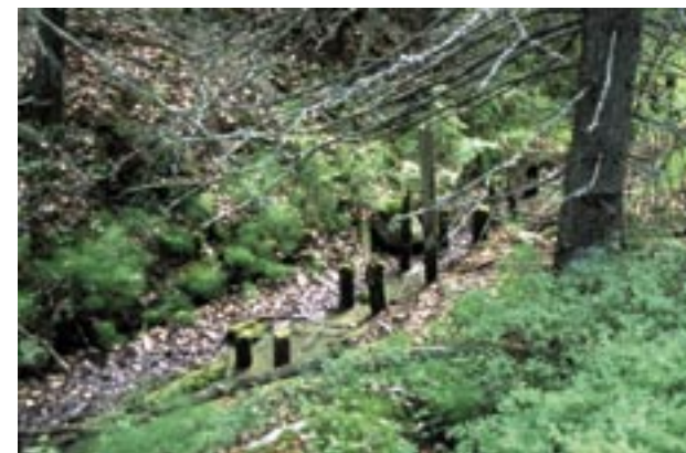
Two photographs showing the construction of canal
