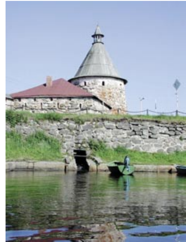
The other end of the water supply tunnel where it enters the dry dock.
