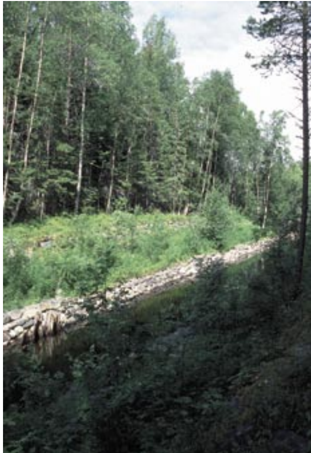
Canal K10 was built around 1900. The excavation work was around eight metres deep and its sides are terraced to make them stronger.
